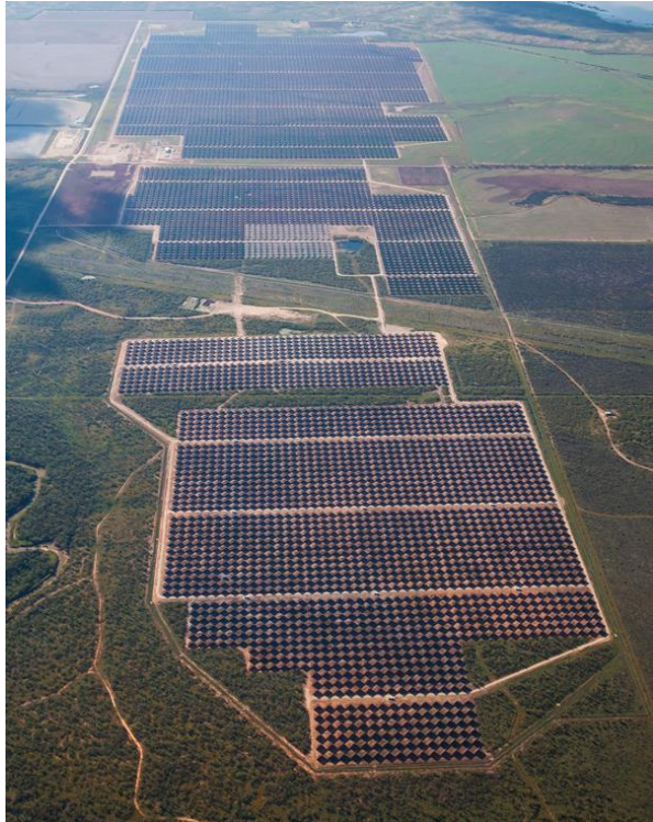
Alamo 7 Solar Farm 106.4 MW – Haskell, Texas
